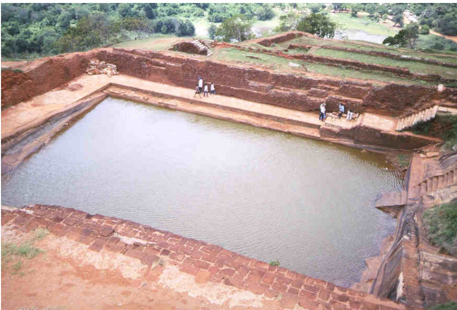
Figure 1: Sigiriya, Sri Lanka. This reservoir cut into the rock was used centuries ago to hold harvested rainwater. ©Practical Action
