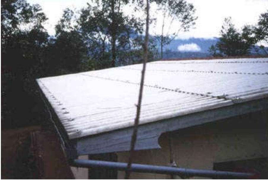
Figure 4: A typical corrugated iron sheet roof showing guttering ©Practical Action
