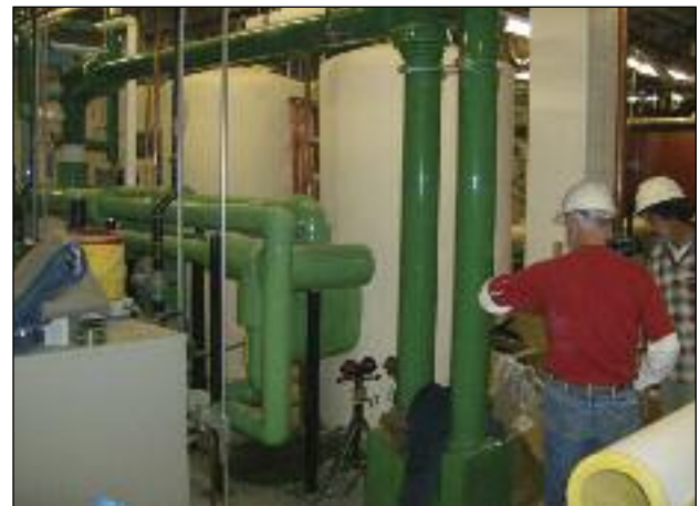
Rainwater storage at the Western Virginia Regional Jail is stored in four 30,000-gallon belowground fiberglass storage tanks. Storage tank selection can be tailored to the site.
