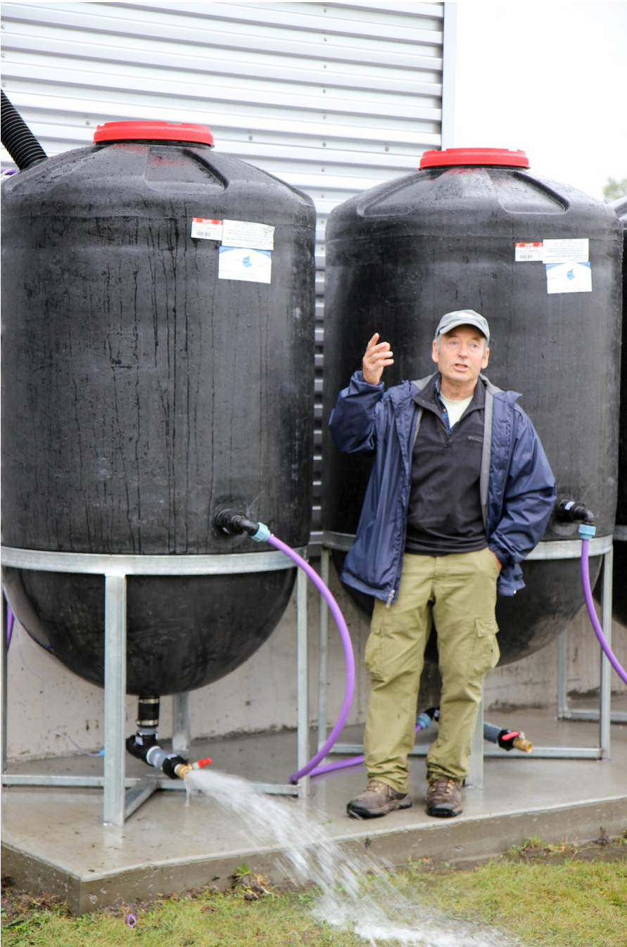
Dr. Amir Yechieli provides a demonstration of the rainwater harvesting system (Courtesy District 113)
